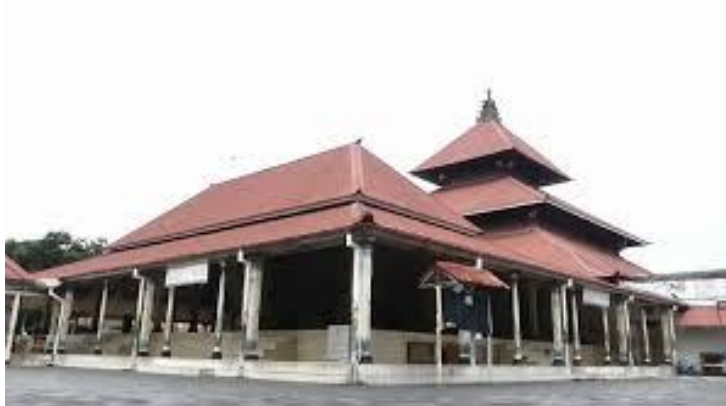
Picture 2. The roof of the Gedhe Kauman mosque is arranged/graded
