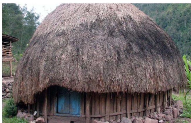
Figure 1. Exterior view of Honai traditional house
